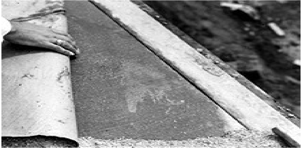
Figure 5: Impervious curing paper for horizontal surfaces.
