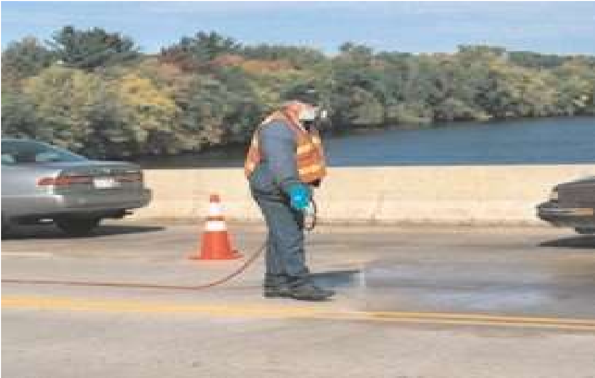
Figure 9: Penetrating sealers help protect reinforcing steel in bridge decks from corrosion due to chloride infiltration without reducing surface friction.
